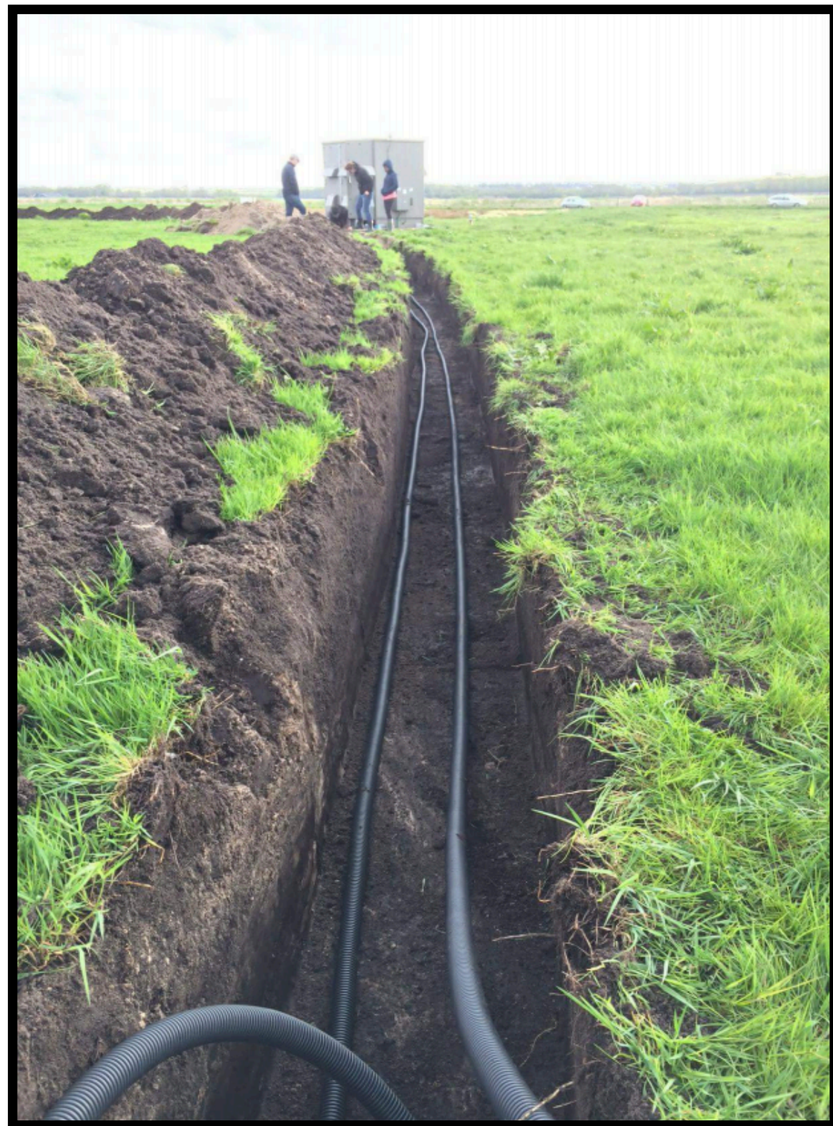
Coax cables for signal and HV
